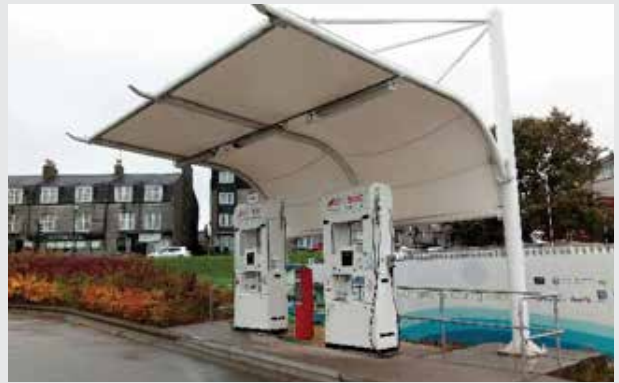
Kitty Brewster Hydrogen Refuelling Station – Aberdeen City
