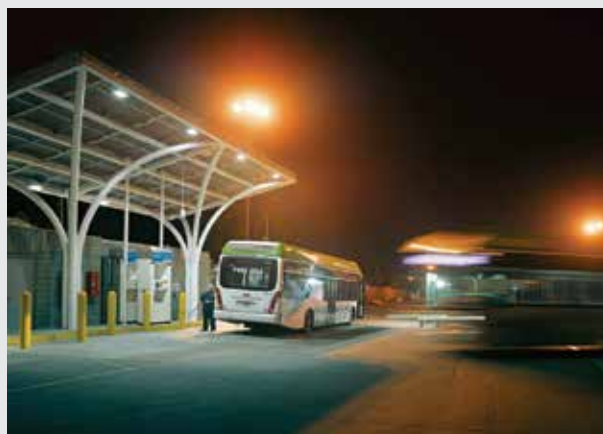
H2 Aberdeen's refuelling station at Kittybrewster
