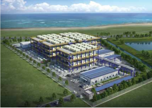
Hanwha Energy and Korea East-West Power have started construction on the world's first 50 MW hydrogen fuel cell power plant. The plant is expected to cover over 20,000 square meters and provide 40,000MWh of energy per year, enough to power 17,000 thousand households. Construction is scheduled to be finished by 2020.
